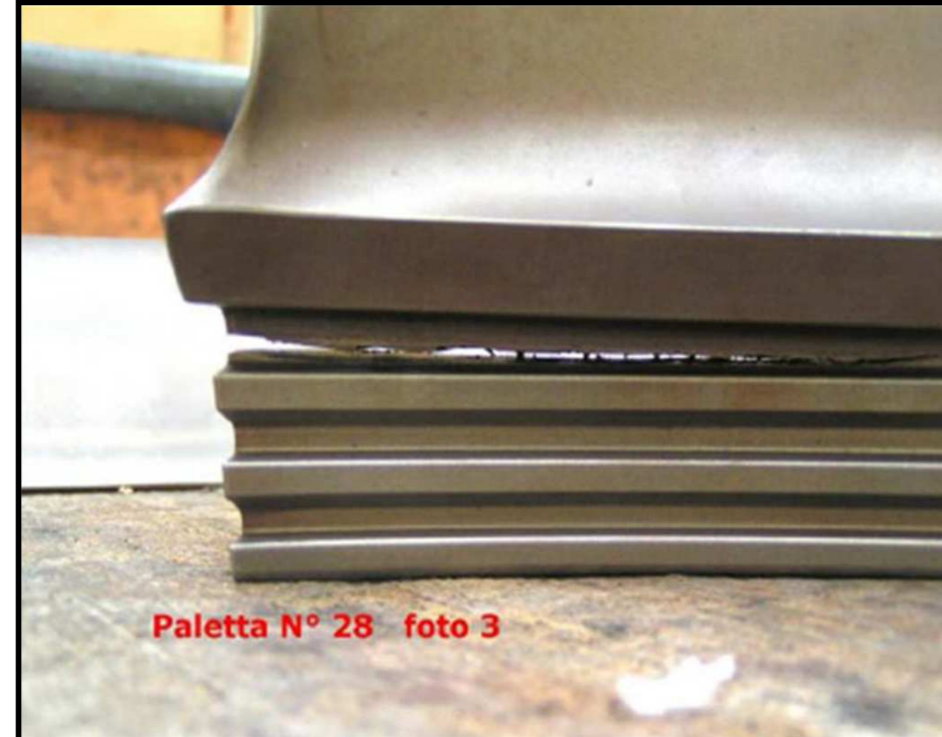
Crack developing in the fir tree root of the first blade of the pack of 8 blades.
